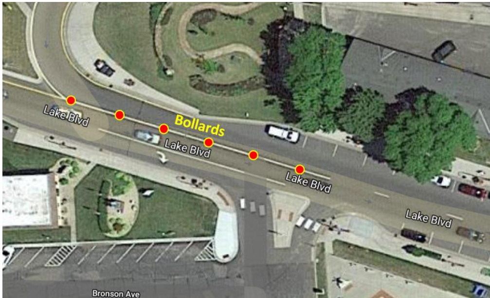
Figure 3 – Bollards on Lake Boulevard at Linden Street
